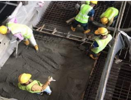
c) Concreting process
