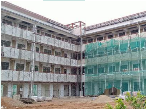
d) Full modular component installation at the site
