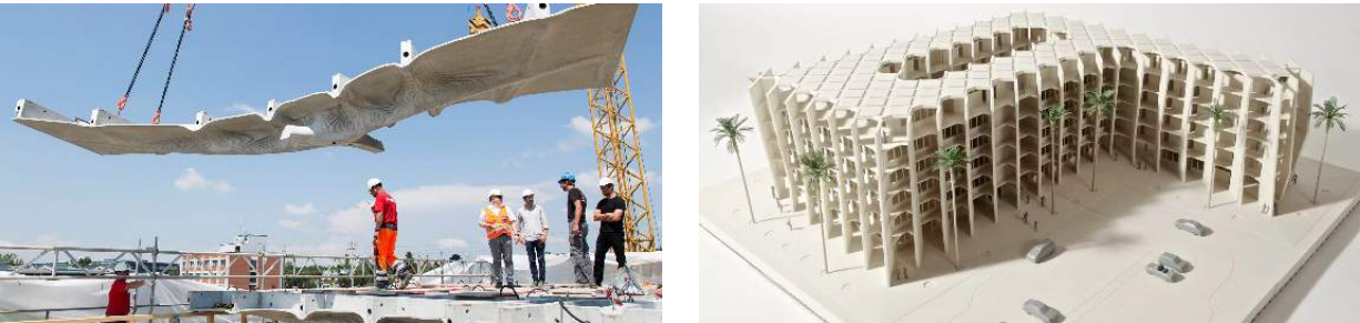
Figure 4.11 3D printed formwork for smart slab (left) and 3D printing for architectural models (right).
