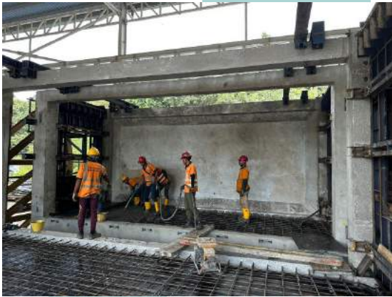
a) Component casting at the factory
