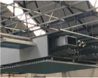
c) Prefabricated MEP module; horizontal module (left), vertical riser module (centre) and plant module (right)
