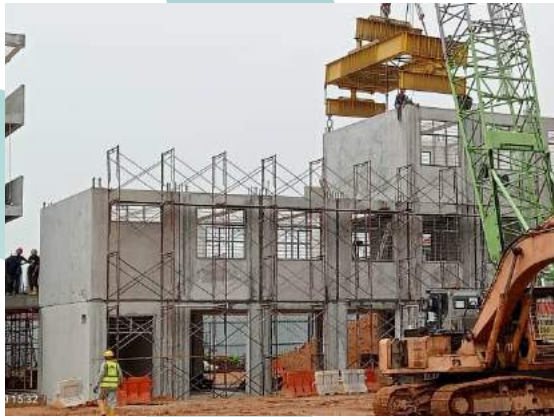
b) Component lifting and installation at the site
