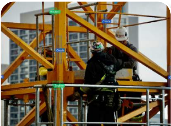
(c) Asset inspection
