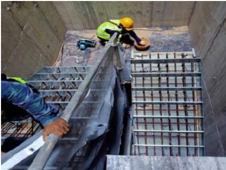
b) Installation of staircase module at the site
