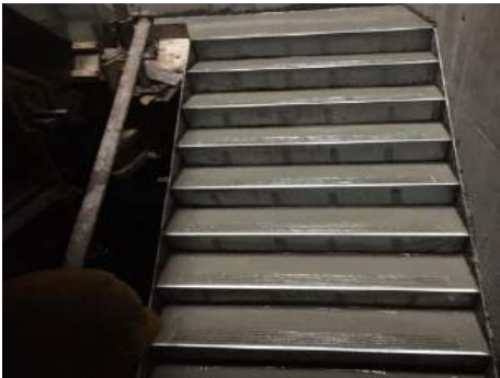
d) Finished staircase
