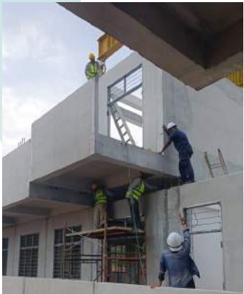
c) Component installation at the site
