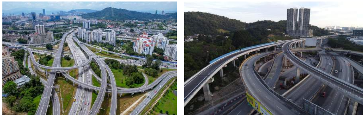
Figure 5.28 The SUKE Elevated Expressway: Aerial View of Hillview Interchange, Ulu Kelang
