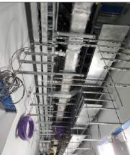
d) Prefabricated modular support completed with MEP
