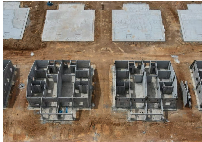
The HCPS IBS Technology is the only one in Malaysia that emulates a monolithic multi-box and modular shear keys system.
