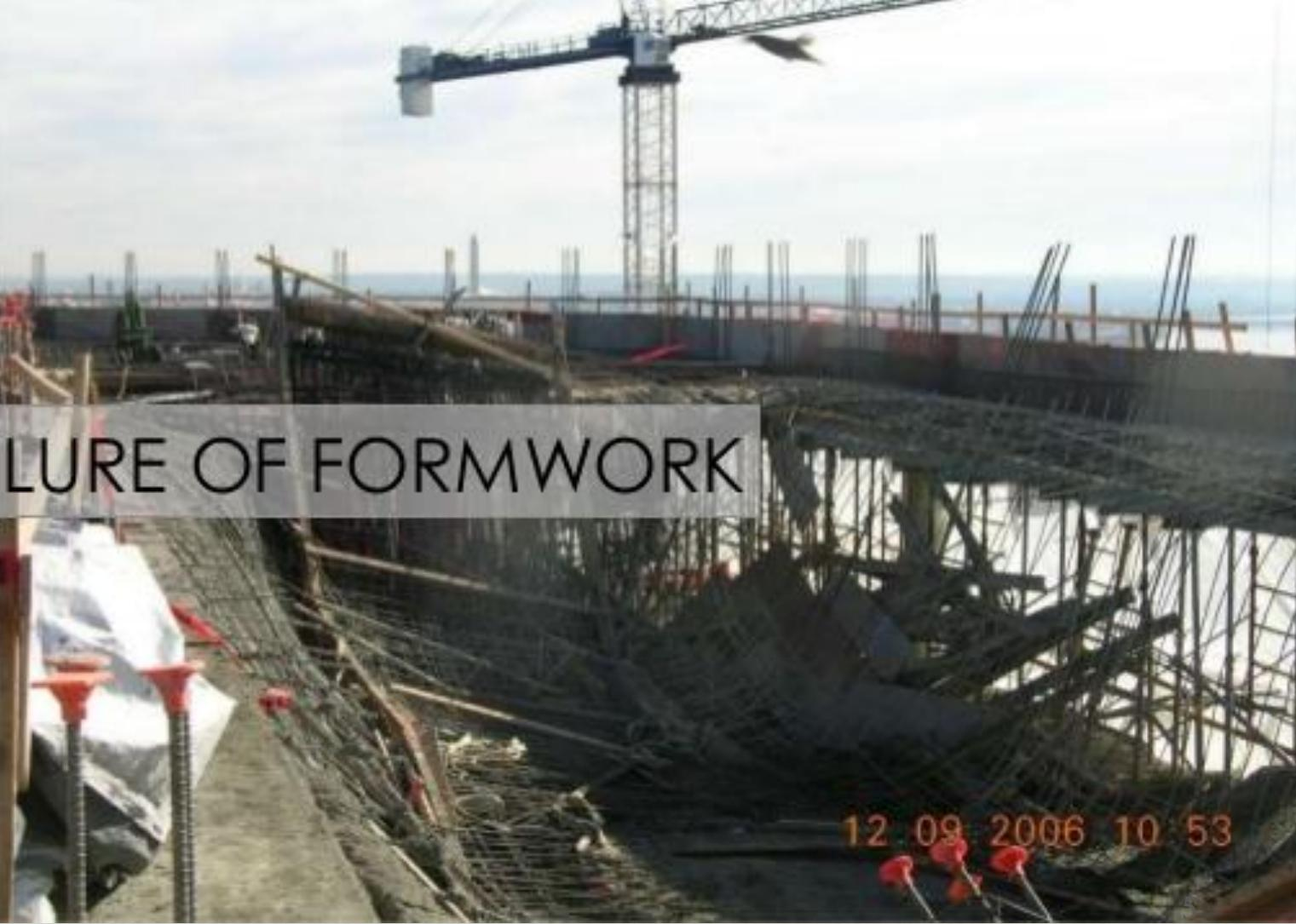
A photograph of a construction site showing a large-scale concrete pour. A section of the wooden formwork has collapsed, causing concrete to spill onto the rebar below. A tower crane is visible in the background. A white arrow points from the left towards the collapsed formwork.
