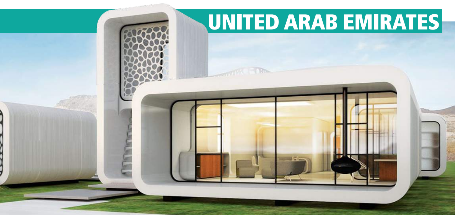
Part of Dubai's 'Museum of the Future', the 185.8-square metre fully functional building will be the world's first 3D printed office. ▲
