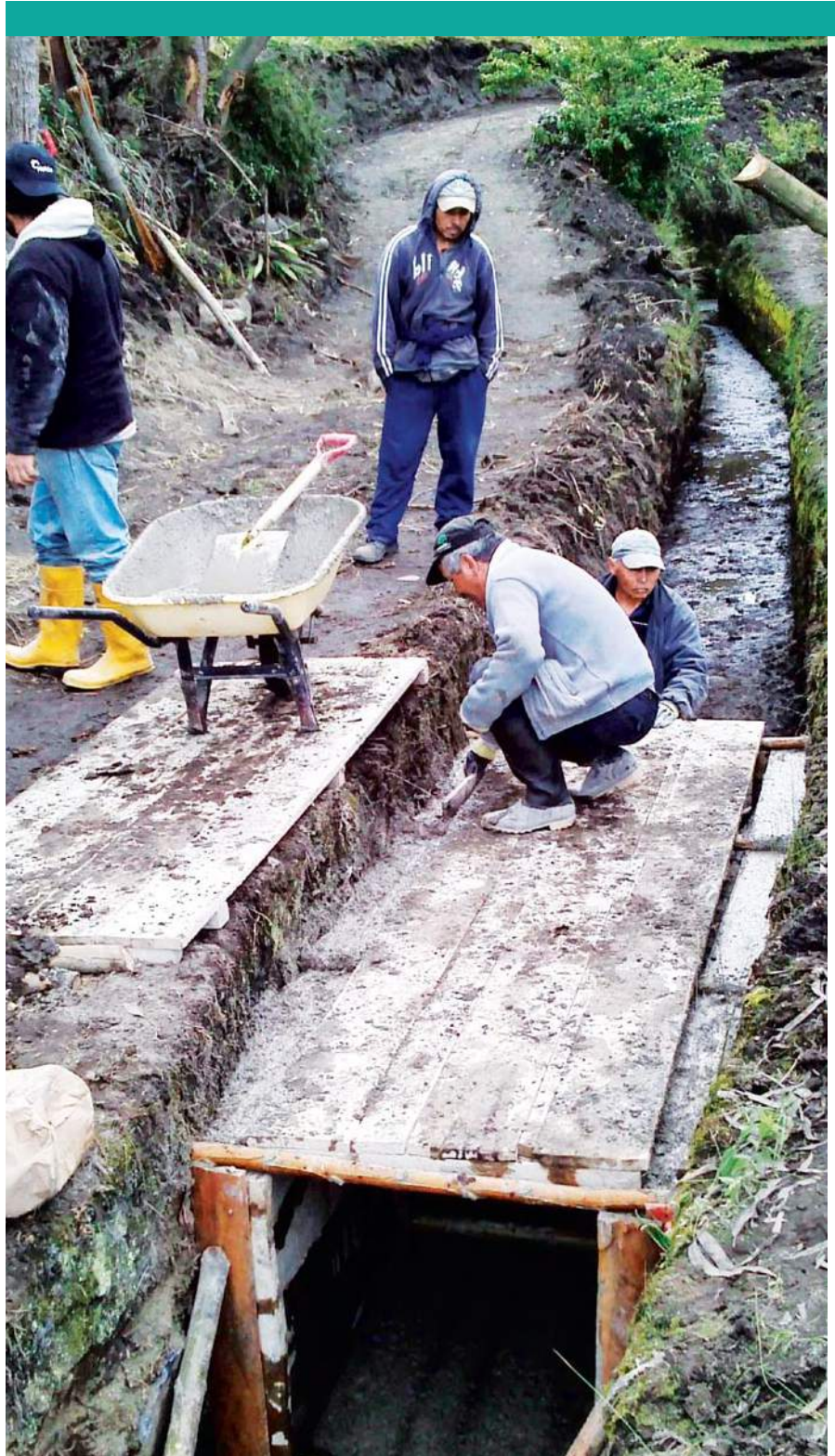
▲ Microbiologist Hendrik Jonkers and volunteers apply self-healing concrete to Ecuador's Cruzsacha canal and irrigation system, which supplies water to 7 communities and more than 400 families.
