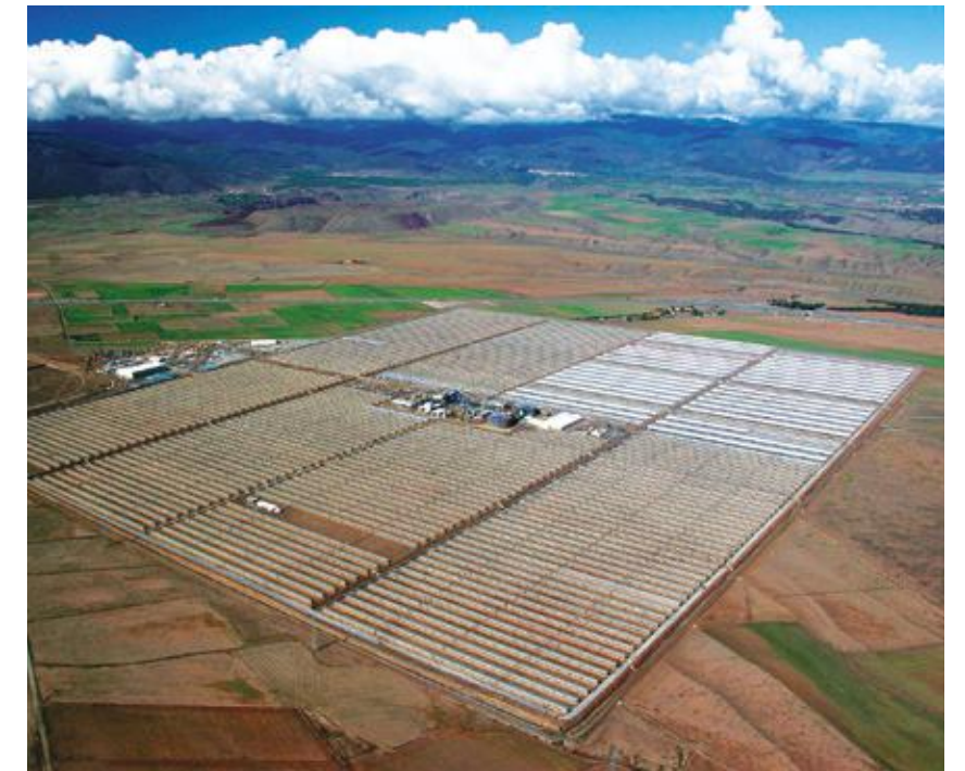
The Andasol solar power station in Guadix, Spain. Its thermal storage system absorbs the sun's heat and stores it in a molten salt mixture for future use. When the storage system is fully loaded, the stored heat can power a turbine to produce about 7.5 hours of electricity, during the evening or overcast days.
