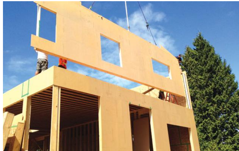
▲ Through the use of industrialised building systems (IBS) where building components are manufactured off-site and then assembled on-site, contractors and sub-contractors can reduce waste and attain greater sustainability.
