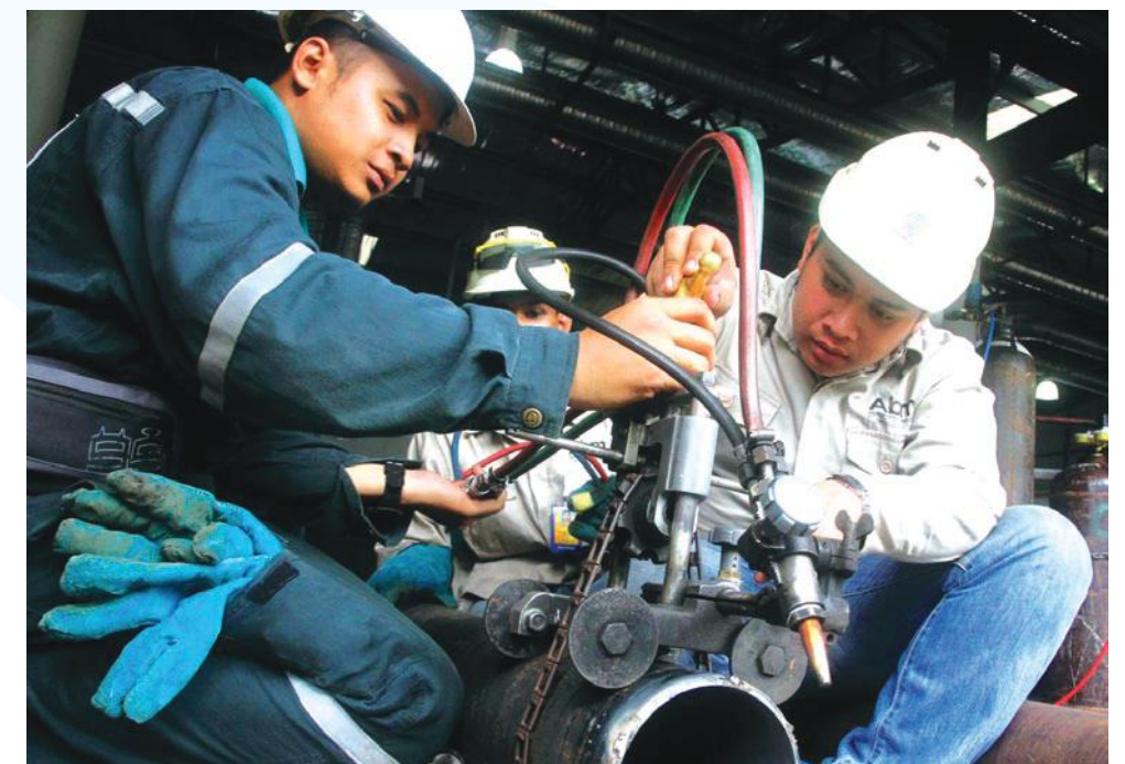
Shahrul Zaimir Nor Zamberi (left), Habitat Technician and graduate of the ABM Eastern Malaysia monitors a welding procedure. ▲
