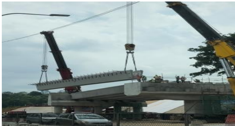
Figure 6: Elevated highway beam installation across public road
