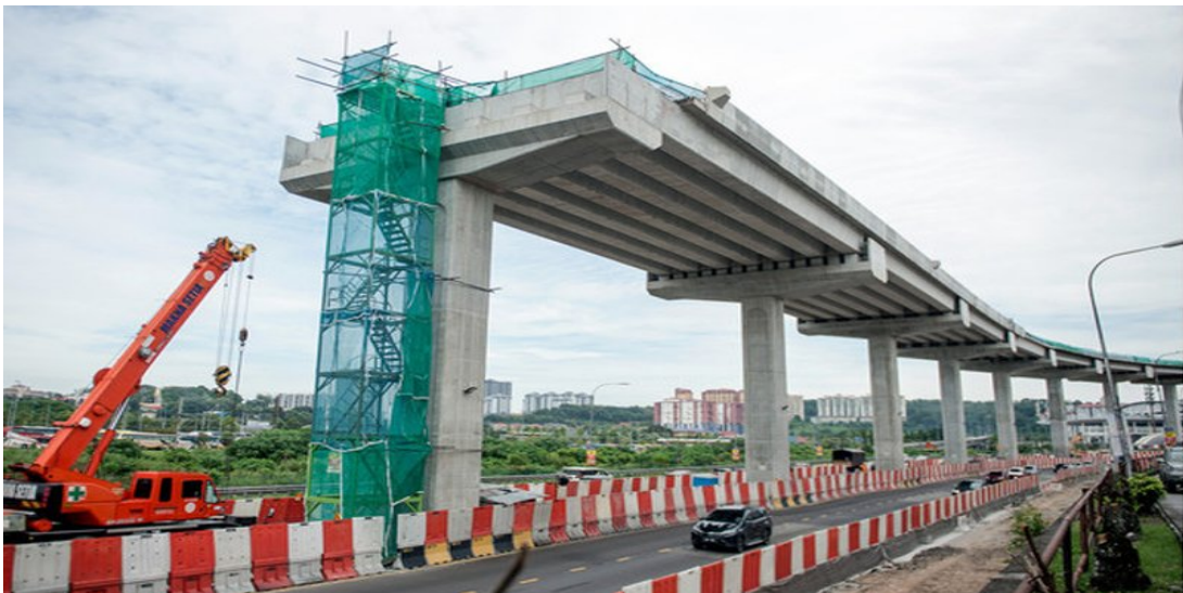
Figure 1: Scaffold and machinery adjacent to live traffic
