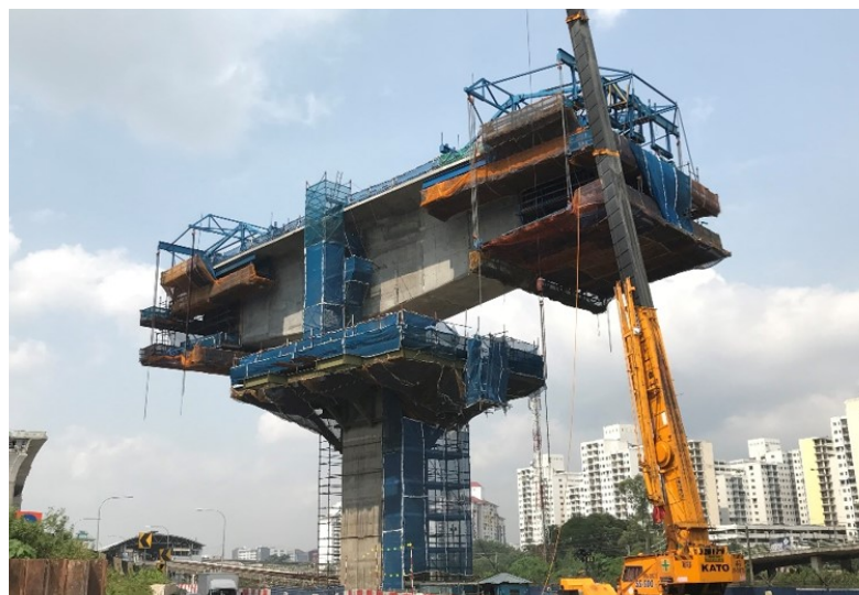
Figure 7: Segmental Box Girder under construction in the middle of the roadway with lifting crane
