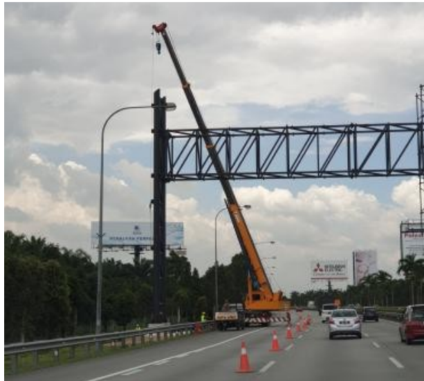
Figure 8: Billboard gantry frame structure installation across public highway
