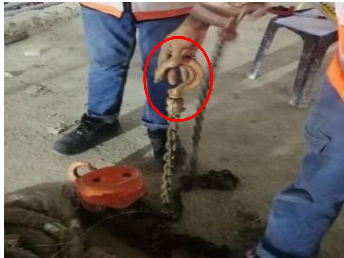
Figure 12: Hoisting without safety latch
