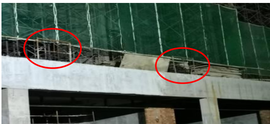
Figure 14: Unused and unsecured scaffold frames, plywood and timber formworks stored at open edge of building perimeter
