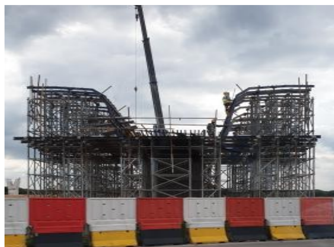
Figure 10: Falsework installation for elevated highway
