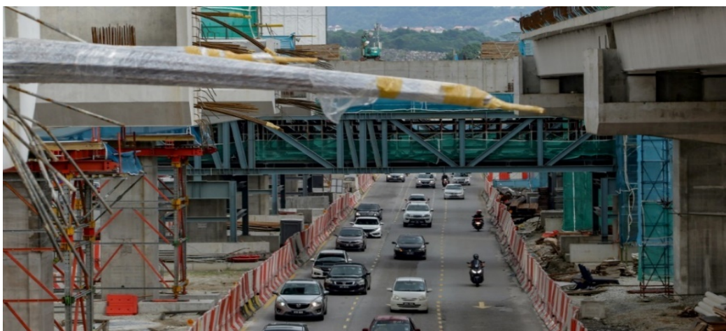
Figure 3: Link bridge construction above live traffic
