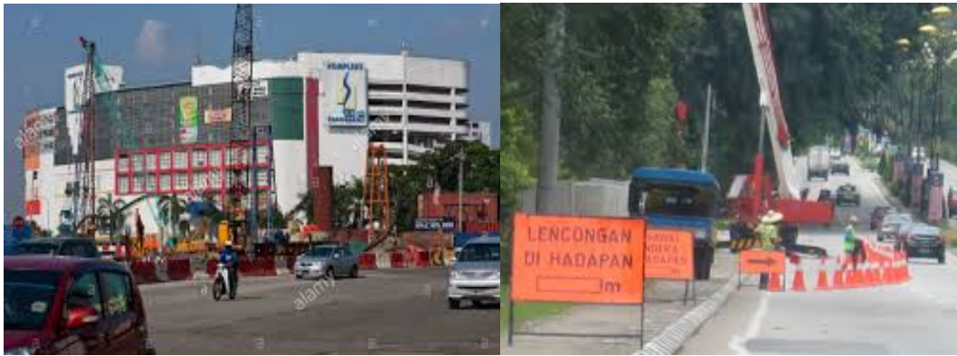
Figure 2: Crane operation adjacent to live traffic
