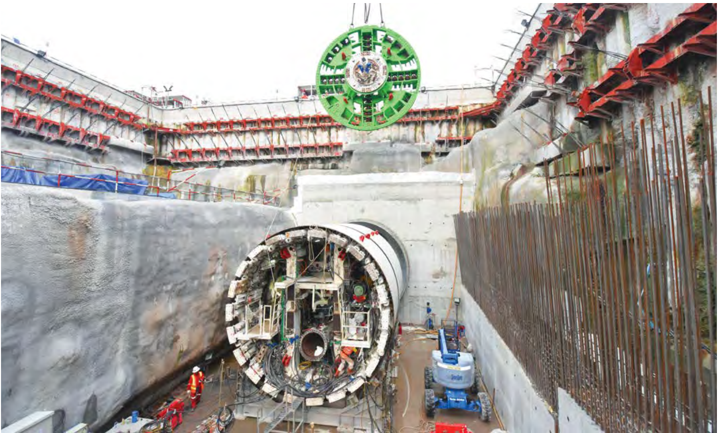
A tunnel boring machine being assembled at an underground station's launch shaft. Tunnelling works couldn't cease during the first Movement Control Order, hence work went on carefully with additional Covid-19 prevention SOPs and safety measures in place. Photo credits: MMC Gamuda
