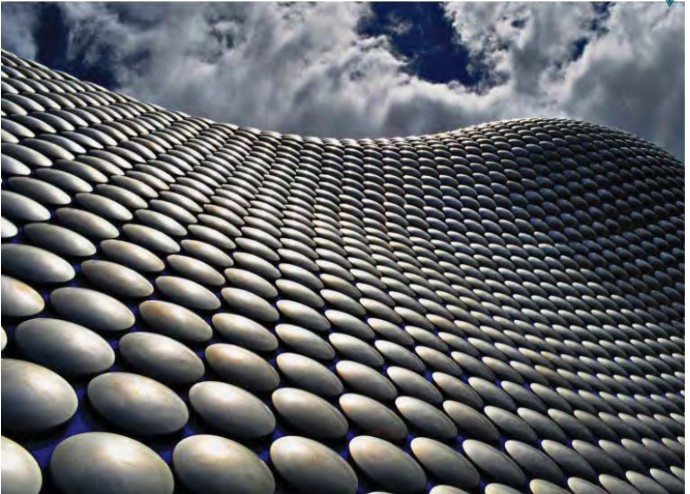
Aluminium discs used as cladding on a building
