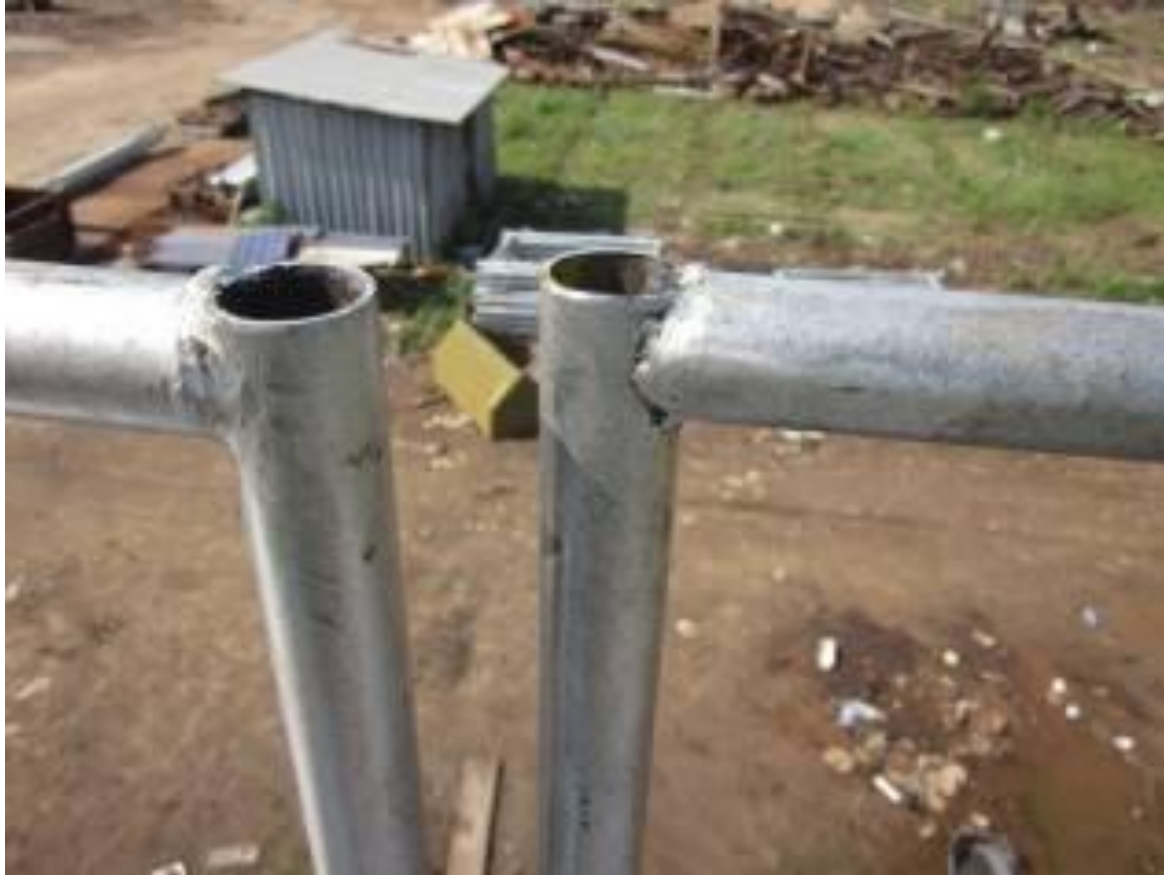
Coupler not installed
