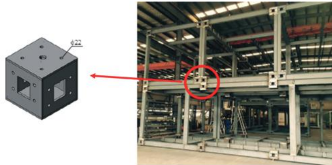
Figure 3.12: Steel bracket connection welded to corner column
