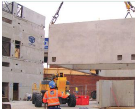
Figure 3.31: Example of block-outs for through bolt connections are seen along module edges
