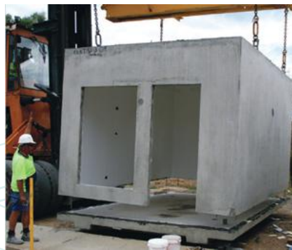
Figure 3.29: Example simple gravity dowel connections on grout pad
