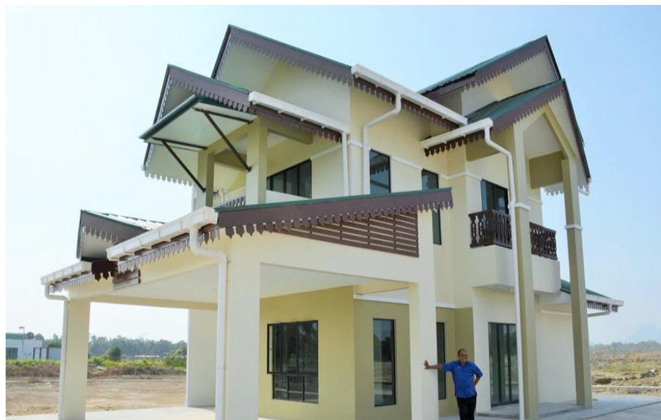
Figure 4.5. Darul Hana two-storey house
