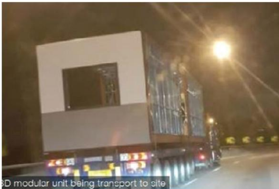
3D modular unit being transport to site
